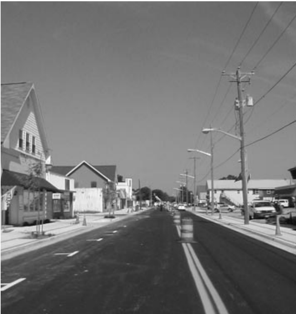
Crews Remove Downtown Exmore's Utility Poles
