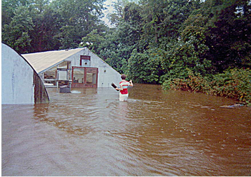
Figure 6: Greenhouse flooded in the Town of Bloxom on September 3, 2003. Photo by Franklin Kreisl
