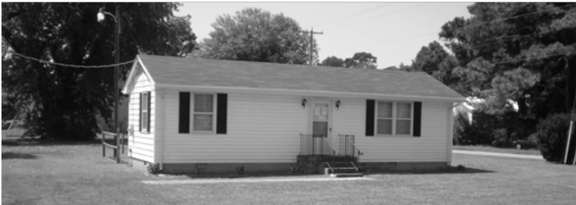
Figure 3: The Keller Town Office is at risk from storm water flooding and wind damage. Photo by Curt Smith
